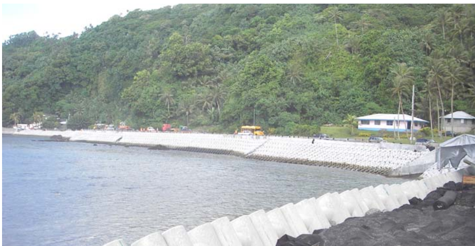
Fig. 21. Erosion control structures such as this seawall in American Samoa can effectively protect coastal infrastructure and development, but are expensive to maintain, and often lead to the conversion of the existing coastal ecosystem into deepwater habitat (photo by E. Gilman).
